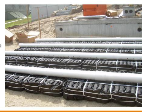
Soil Absorption System – Bottomless Sand Filter (BSF)
