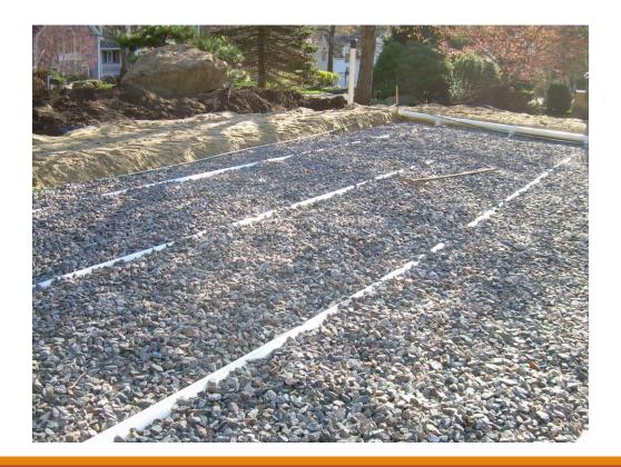
Soil absorption system chambers, pits or galleries -
