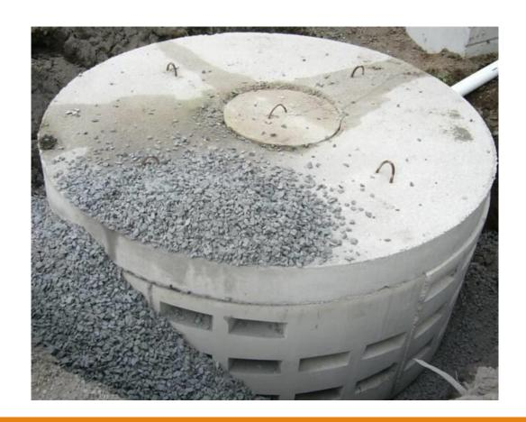
Soil absorption system aggregate -
